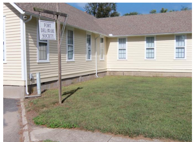
33 Staff Lane Freshly Painted
